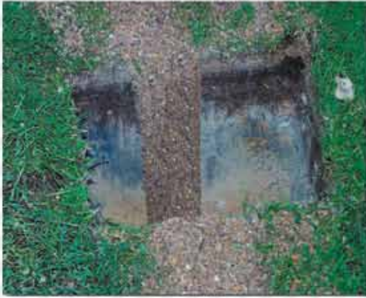
CUTAWAY SECTION OF TOPDRAIN MATRIX
